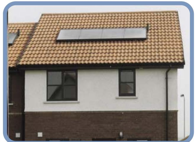
Figure 7: Solar thermal panel
