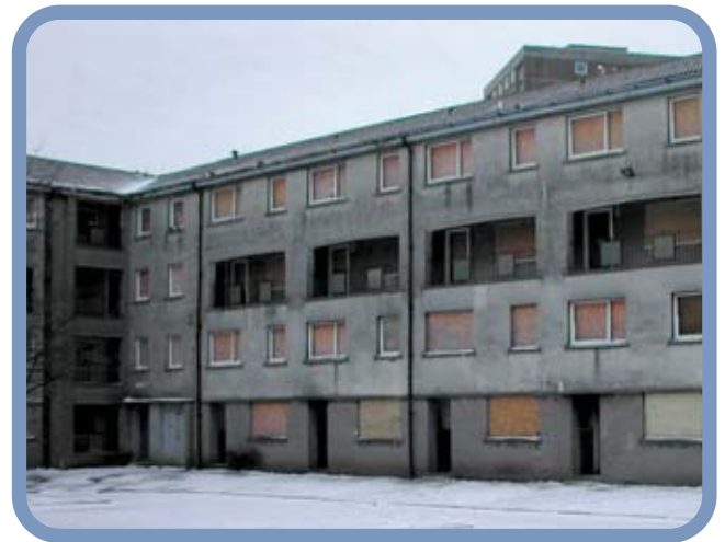
Figure 1: Flats before improvement
