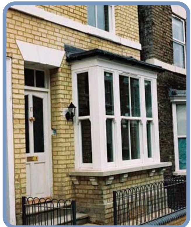
Figure 6: Front view after improvement
