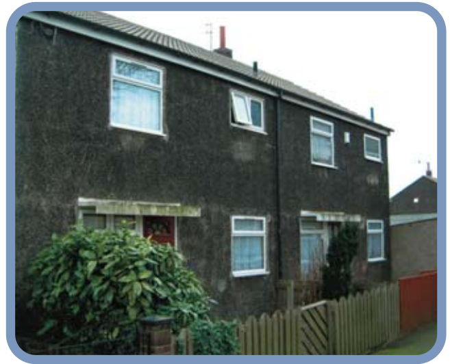
Figure 8: Houses before refurbishment
