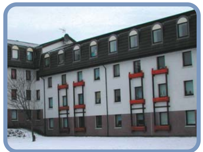
Figure 2: Flats after improvement
