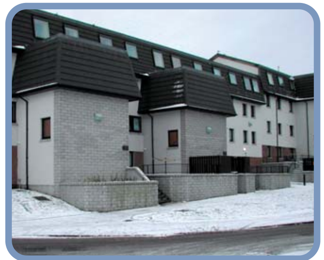
Figure 4: Flats after improvement
