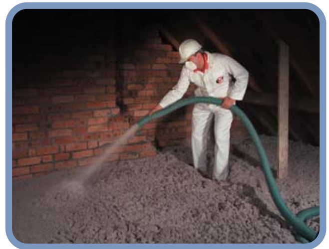
Figure 7: Insulation being blown into loft spaces
