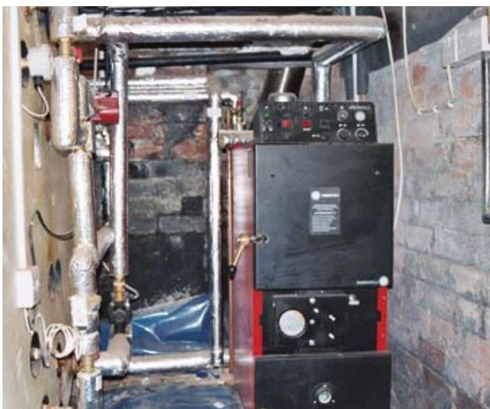
Hybrid system in basement including heat store and log boiler
