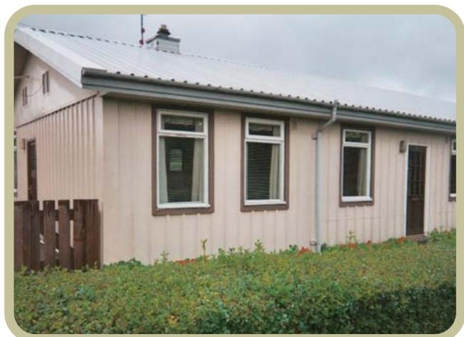
Figure 4: Aluminium-framed property with metal cladding, 1947.
