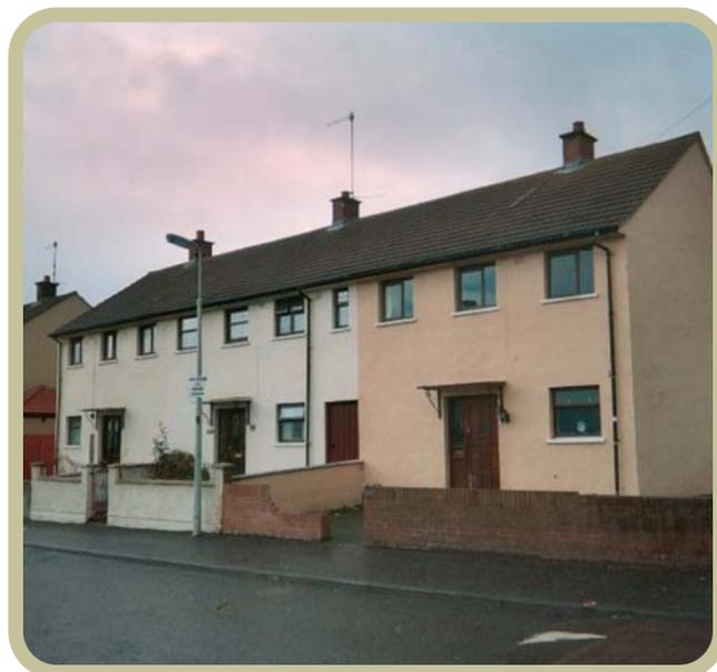
Figure 6: No-fines concrete housing, circa 1951.
