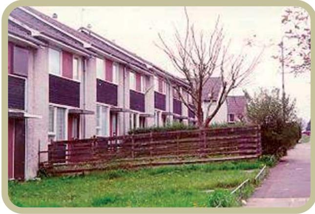
Figure 7: Housing incorporating timber infill panels.
