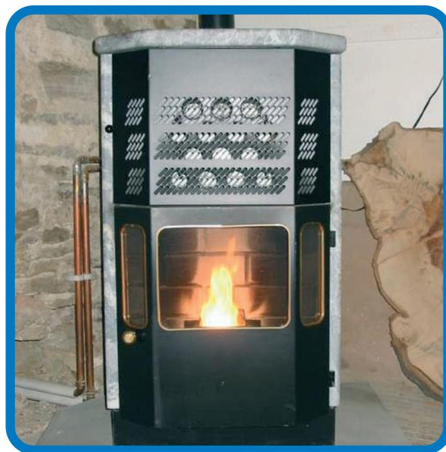
Figure 7: A pellet stove with back boiler (Source: Centre for Sustainable Energy)
