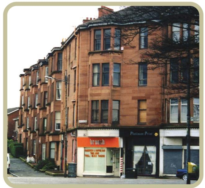
Figure 1: A typical pre-1919 red sandstone tenement
