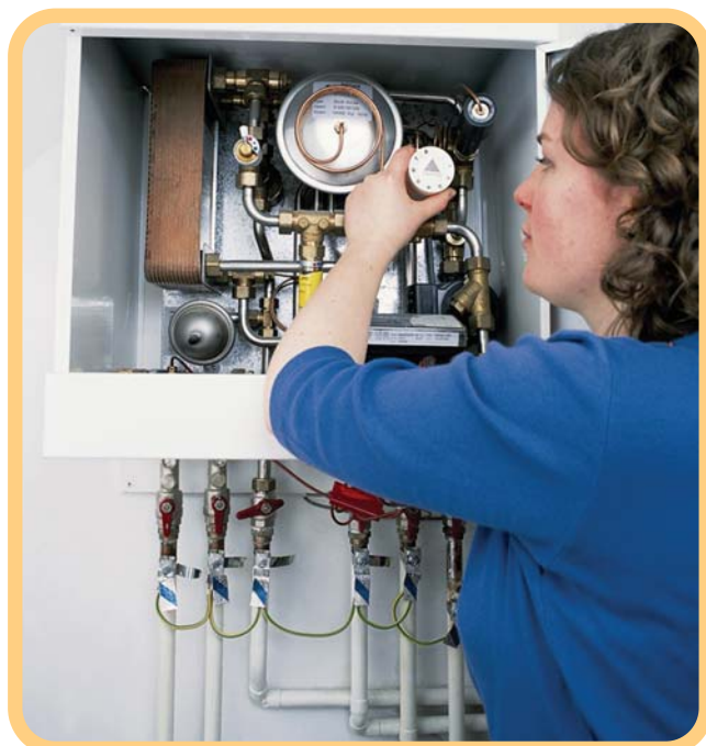
Figure 4: A typical Hydraulic Interface Unit (the connections are similar to those of a conventional gas boiler except that, instead of being connected to a gas main, it is connected to a heat main).
