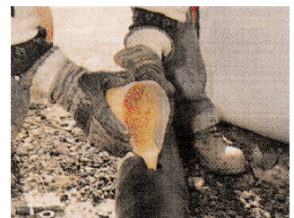
Filling with expanding foam insulation
