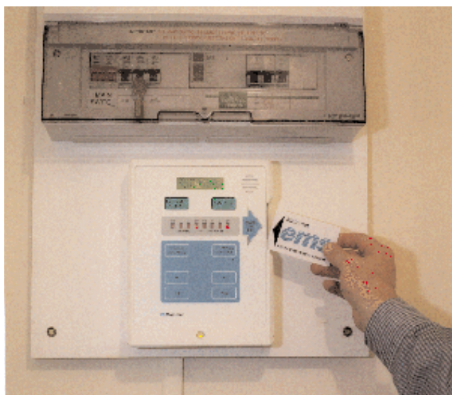
Figure 8 Modern metering systems are very reliable. Administration costs and the risk of non-payment can be minimised through the use of prepayment meters
