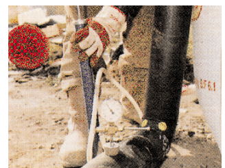
Pressure testing the protective sleeve
