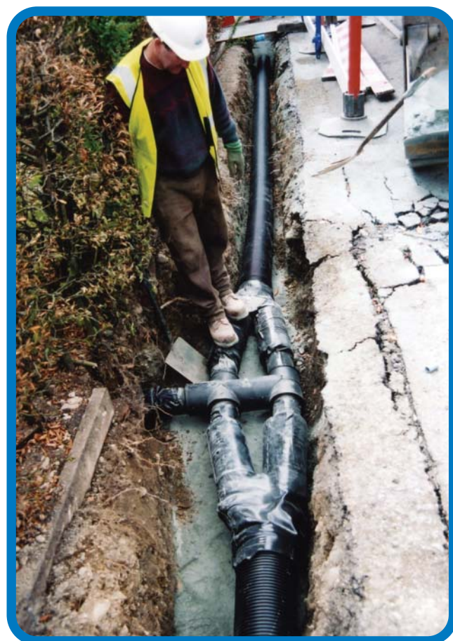
Figure 4: Installation of the heat network
