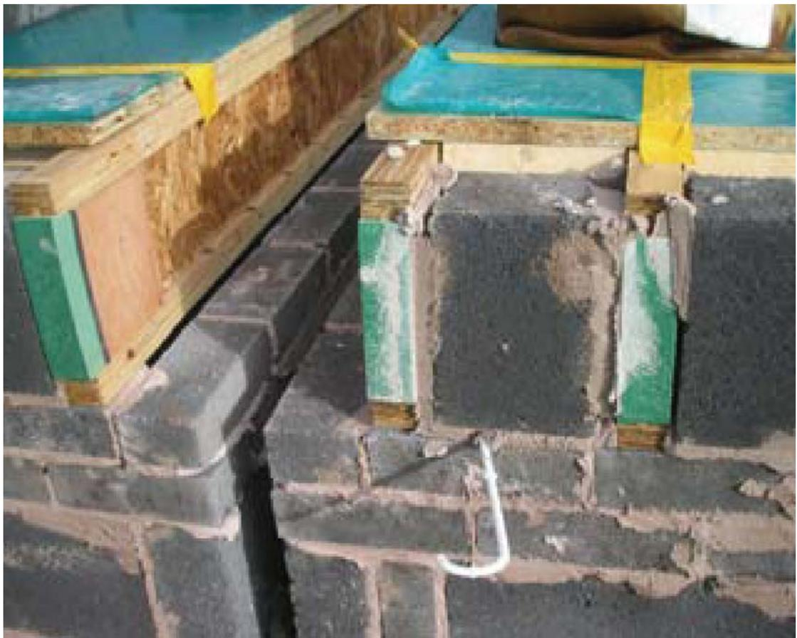
Figure 2: Even if proprietary systems are used to achieve airtightness when joist ends are built into the masonry, the potential for heat losses from thermal bridging or uncontrolled air leakage remains. Blocks have to be cut to fit between the joists, gaps have to be pointed up with mortar. (Photo from Stamford Brook report on airtightness – courtesy of Malcolm Bell, Leeds Met University.)
