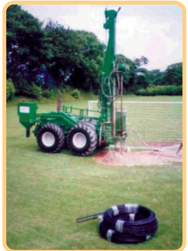
A typical drilling rig © GeoScience 2002
