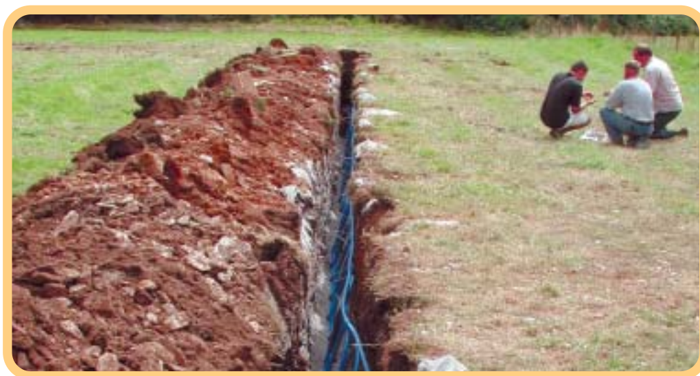
Trench and 'slinky' © GeoScience 2002
