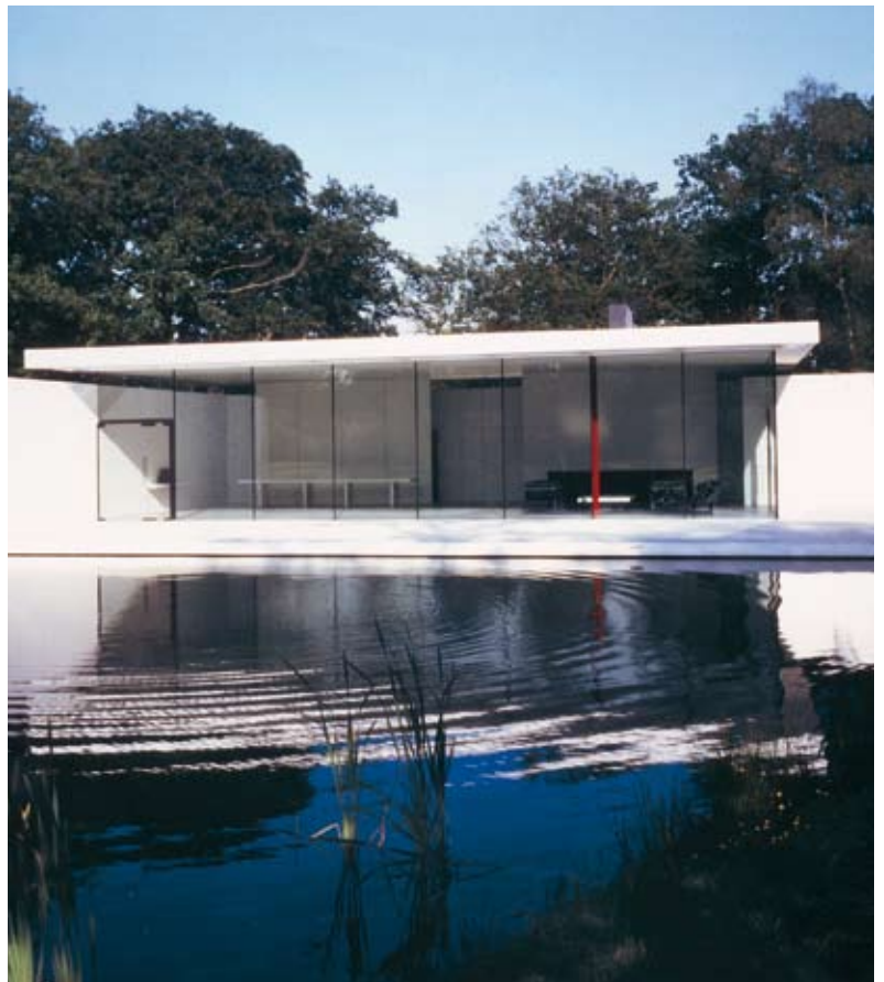
Figure 2 Skywood House, Middlesex, by Foster and Partners (photo courtesy of Sto Limited)
