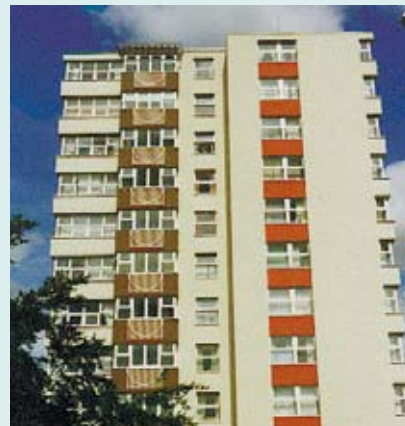
Figure 11 Example of a refurbished high-rise building – Moorfield, by Bristol City Council
