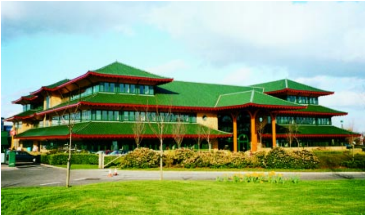
Figure 3 The Body Shop headquarters at Littlehampton has an envelope that acts as the main climatic modifier between the internal and external conditions
