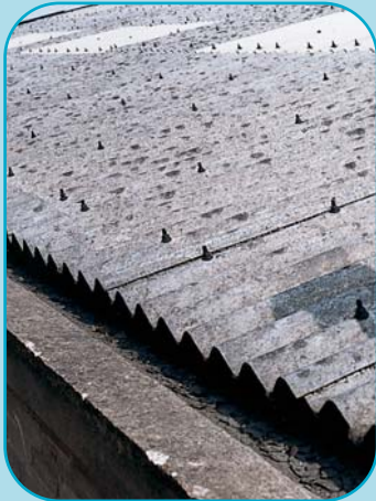
Asbestos cement roof
