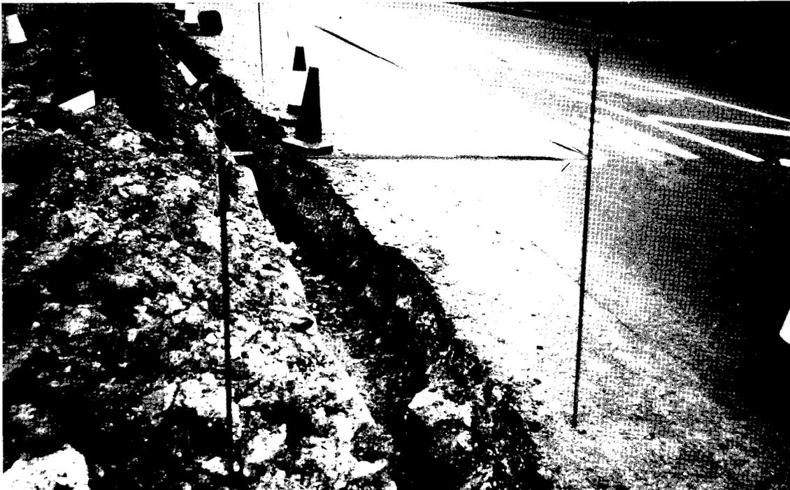
Fig 7 Example of a trial trench dug to find the position of gas service connection pipes
