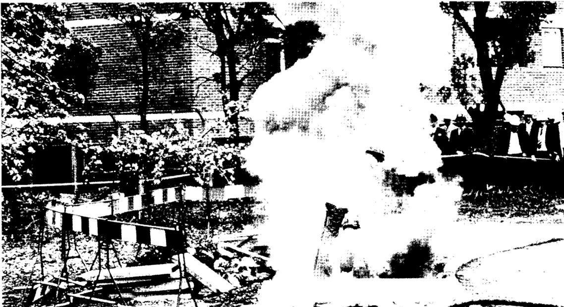
Fig 2 Striking an underground electricity cable can cause serious burn injuries
