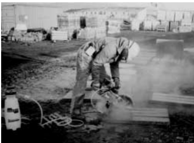
(a) (b) Figure 1 Slab cutting with pressurised portable tank system: (a) without control; (b) with control
