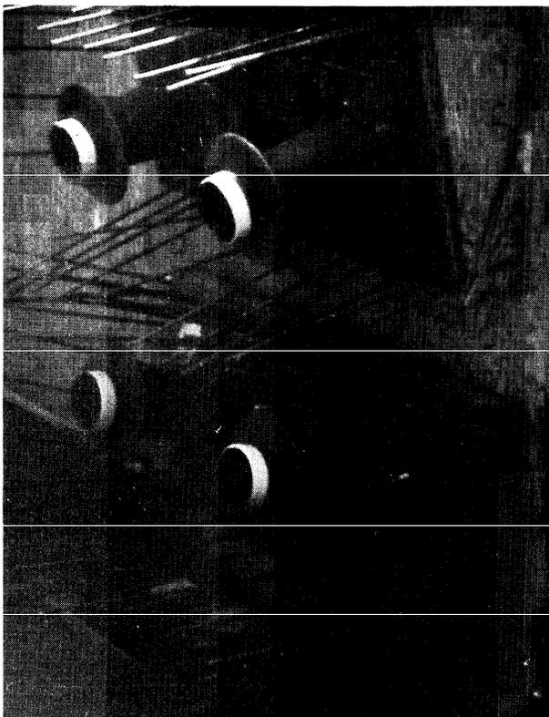
Fig 5 End anchorages after concreting
