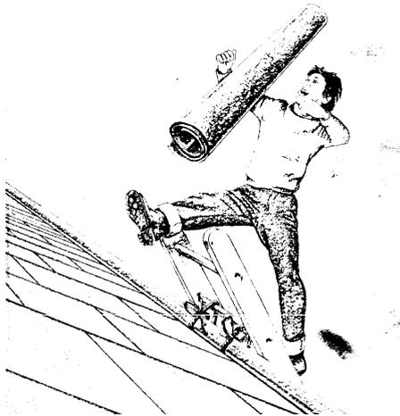
Man carrying a roll of roof felt on his shoulder up a ladder to roof level. Loses control of roll, man and materials fall to ground.
