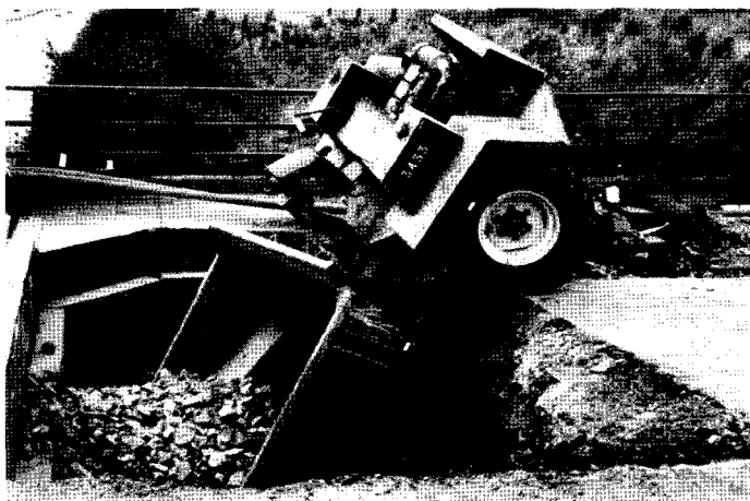
Figure 14 Small site dumper fallen into excavation due to lack of wheel stops
