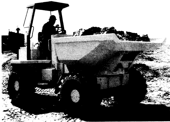
Figure 7 Site dumper with ROPS
