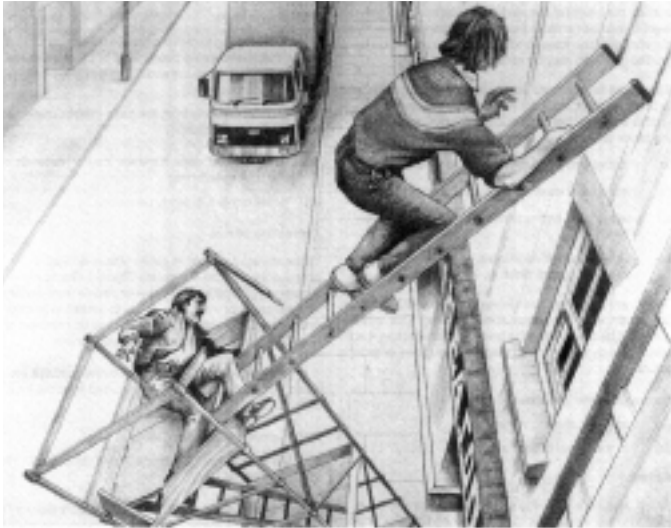
Overloading the top causes this.
