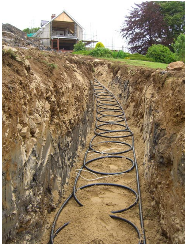
Figure 3 Trench and SLINKY™ © GeoScience
