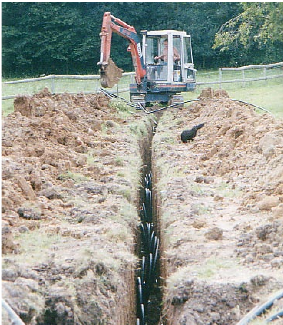
Figure 6 Installation of a vertical Slinky ground collector © Kensa Engineering
