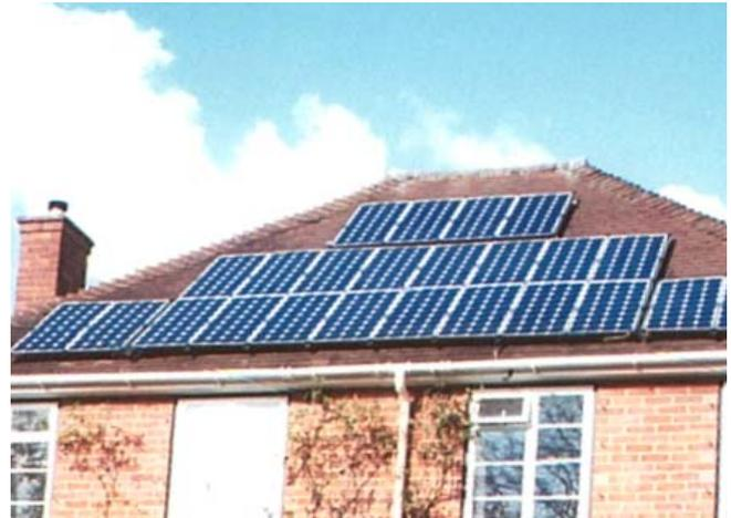
load. In practice, though, there is likely to be considerable resistance to wind flow beneath the modules due to the small gap between the underside of the module and the roof and additional blockage caused by the supporting brackets, fixings and electrical installations which will lead to larger net loads.
