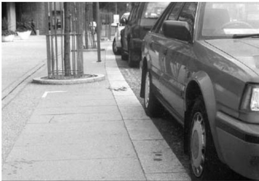
Kerb free level access parking bays with a transfer area defined by surfaces, textures and planting. This avoids the use of painted lines on the road and pavement.
